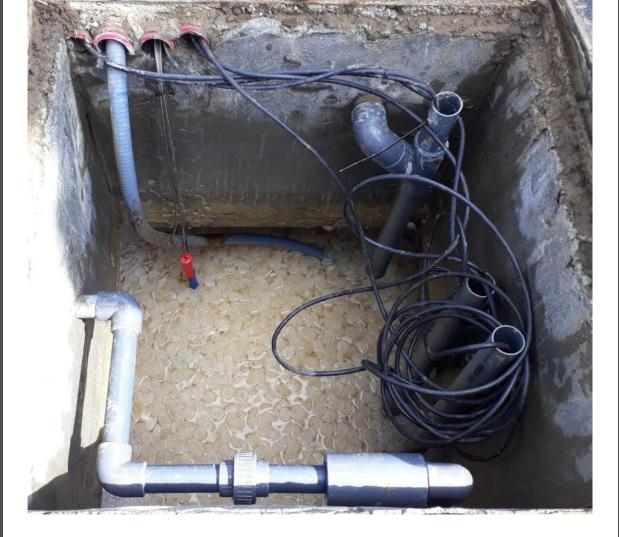
Nitrate removal can be achieved by biological denitrification to nitrogen gas. NuReDrain partner PCS has been intensively testing the Moving Bed Biofilm Reactor (MBBR) filter that uses this principle as working mechanism. A complete and easy to use construction manual of this filter can be downloaded on our project website.
